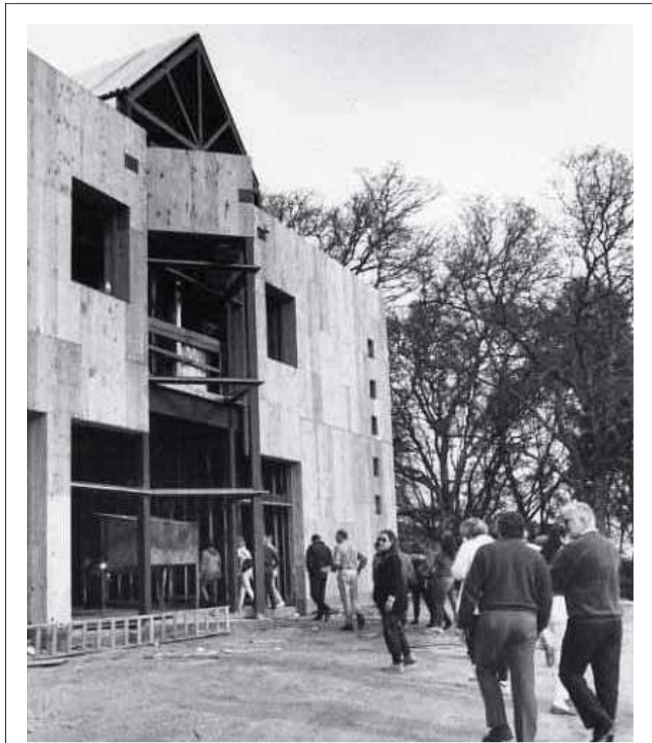
Construction of El Dorado Center - Building B - 1992
